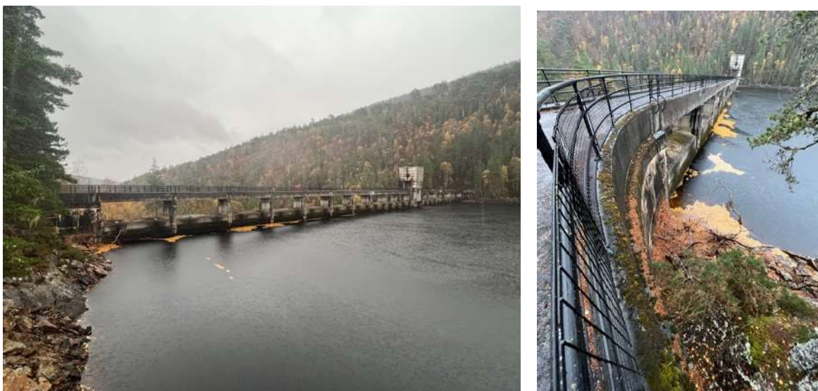
Figure 1 & 2. Beinn a' Mheadhoin Dam, upstream.
